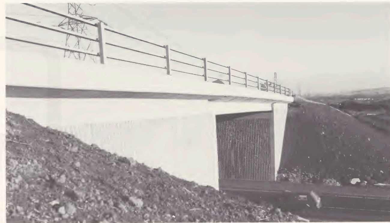
Lasswade Road Bridge
