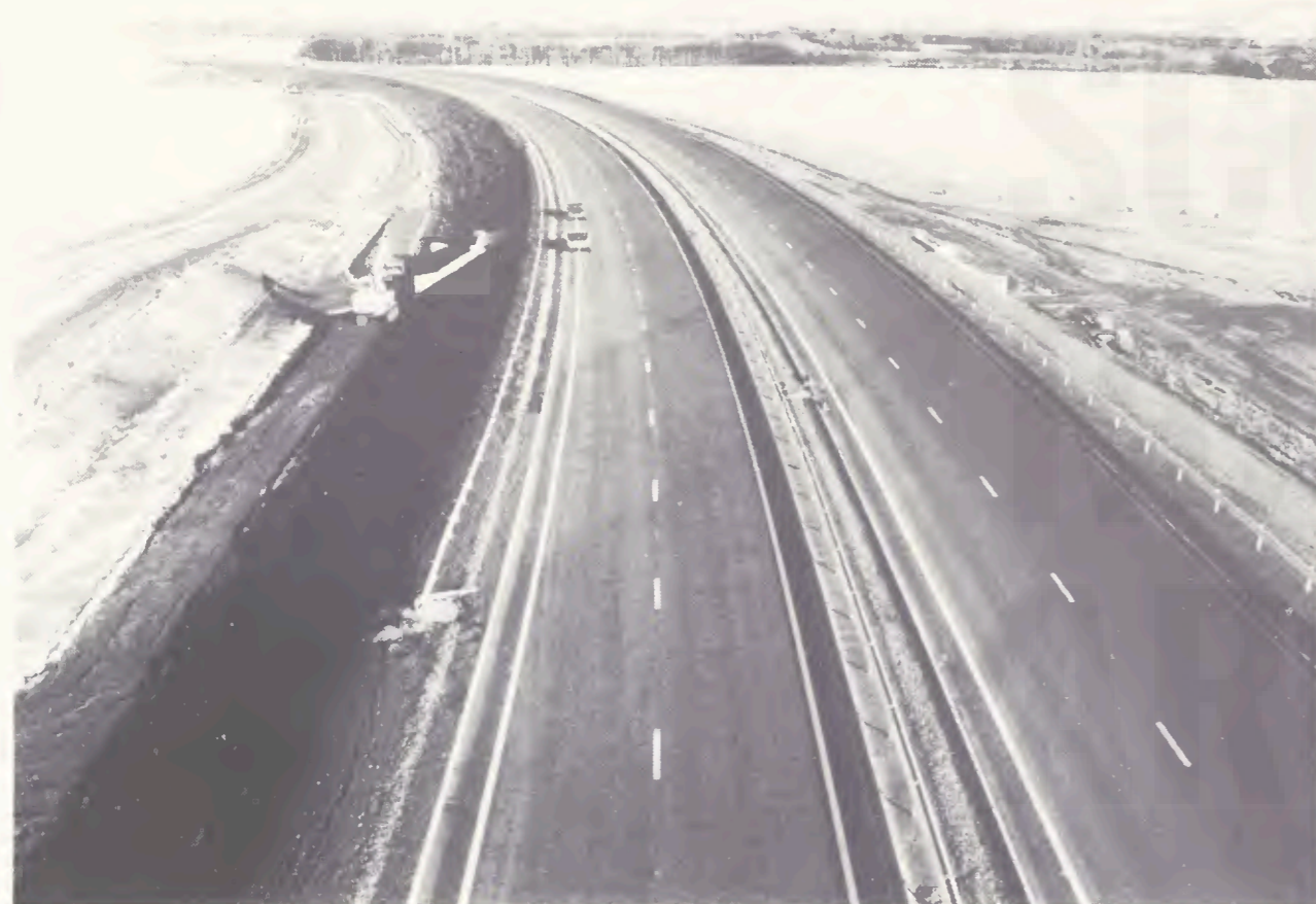
Bypass crossing of Newton Farm Underpass which maintains the Public Right of Way to Newton Church
