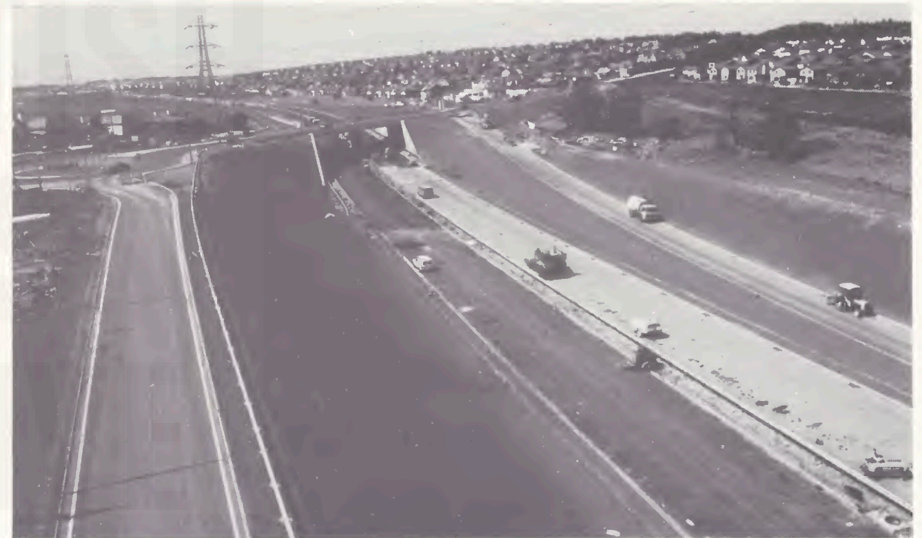
Biggar Road Junction from the East
