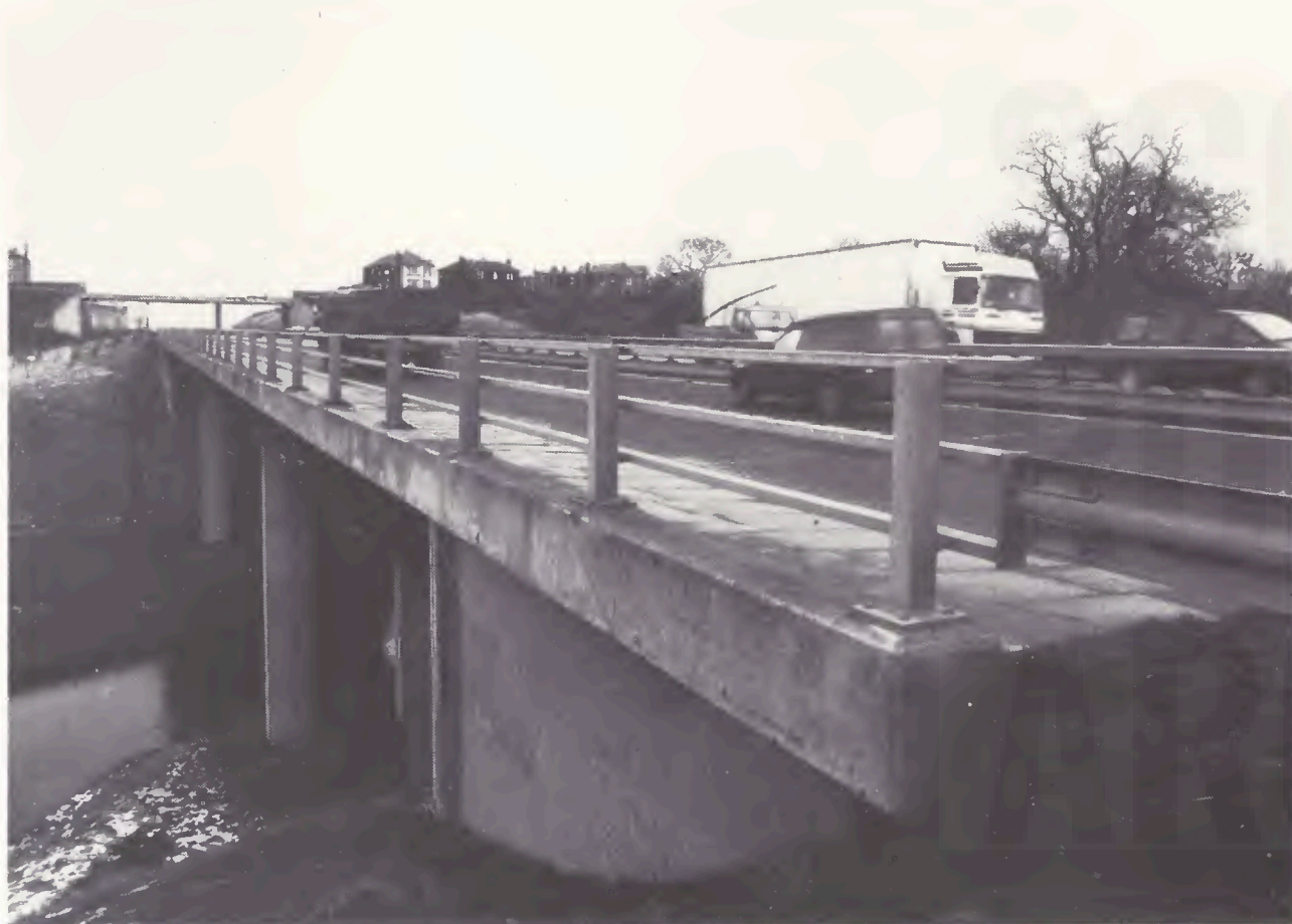
Water of Leith Bridge
