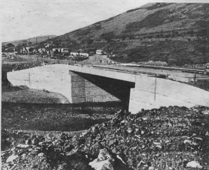
FIG. 6 EVAN WATER BRIDGE.
