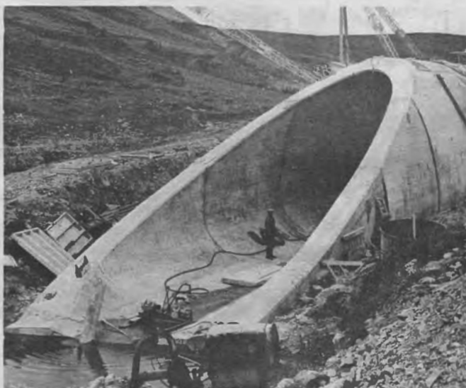
FIG. 3 HARTHOPE CULVERT NORTH.
