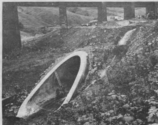
FIG. 4 HARTHOPE CULVERT SOUTH.
