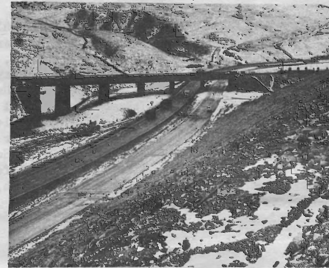
FIG. 1 HARTHOPE VIADUCT LOOKING NORTH.
